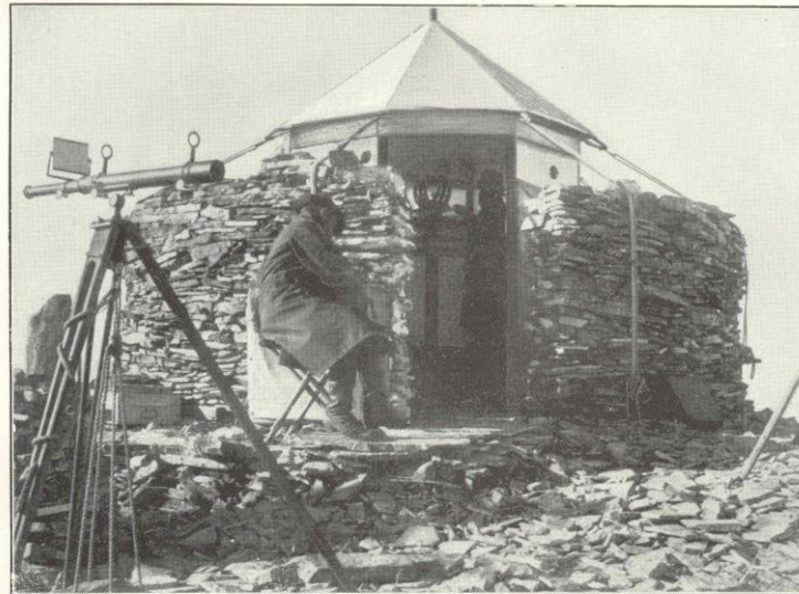
HIGH SUMMIT STATION, TUSHAR MOUNTAIN, UTAH, SHOWING RING WALL AND DOUBLE SHELTER TENT AGAINST STORMS AND RADIATION OF HEAT.
